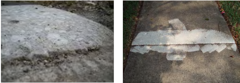
Figure 12: Typical Results from a Grinder
