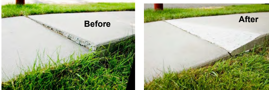
Figure 11: Precision Sidewalk Safety Work Example
