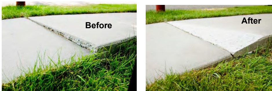
Figure 11: Precision Sidewalk Safety Work Example
