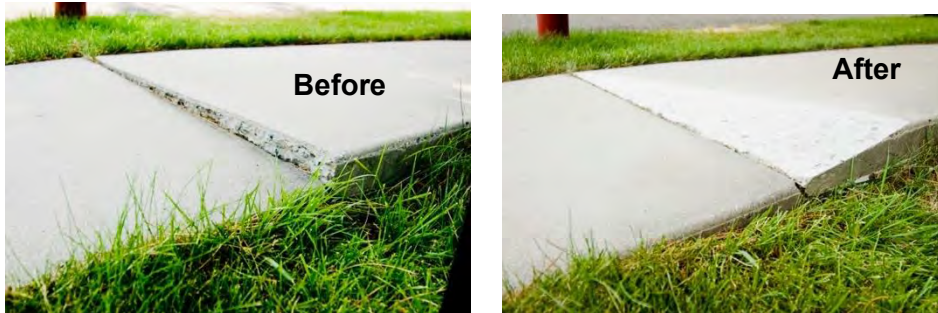
Figure 11: Precision Sidewalk Safety Work Example
