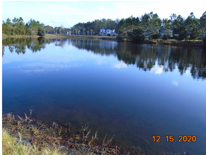
Pond K: Perimeter vegetation is decaying.
