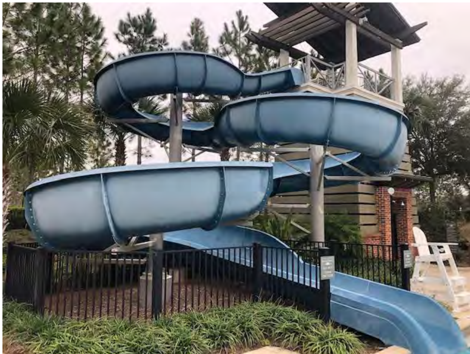
Polish and Wax and Paint Exterior of (1) Open Waterslide. Caulk All Seams.
